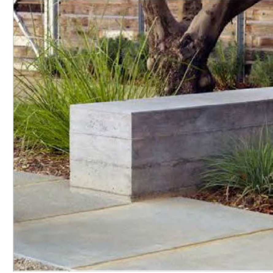
CAST IN PLACE CONCRETE SEAT WALLS
